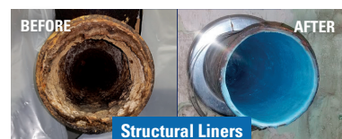
6" Cast Iron Drain Line Before & After Epoxy Lined
