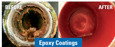
3" Water Main Before & After Epoxy Coated
